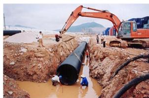
In the ring stiffness classification, there are SN2, SN4, SN8 and SN16 four grades. Usually SN4 and SN8 will be selected. SN8 is preferred for some areas with worse geological condition, e.g. at the Shanghai area, the loading capacity of soil is less and the underground water level is relative higher, so in designing the SN8 plastic pipe is required.
